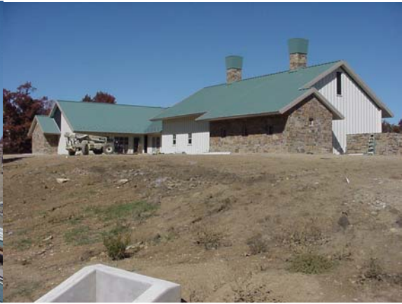
Back entrance (facing S) (classroom wing left, laboratory/office wing right)
