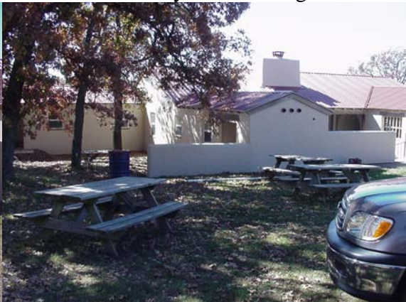
N side of residential structure
